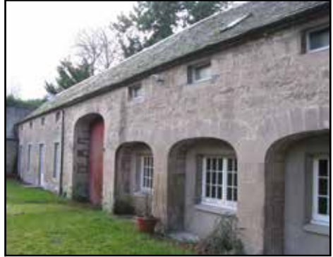
Farm buildings of Newton Court
